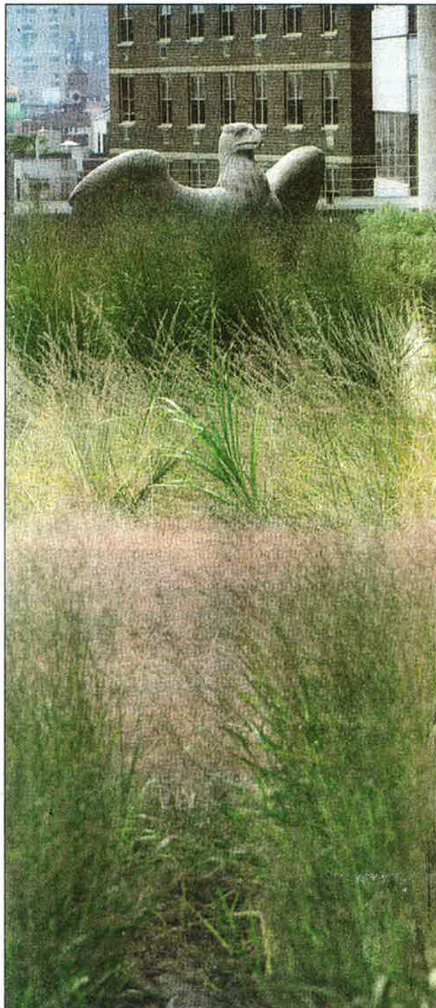
The green roof of 41 Cooper Square, Cooper Union's LEED Platinum building, is adorned with an original eagle from PENN station. The green roof has a water system that irrigates plants and services the building's plumbing.
