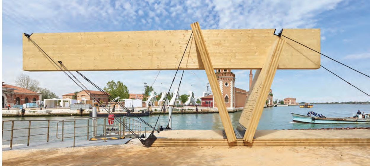
Nader Tehrani's exhibited works included an entry portal and vaporetto stop, made of cross-laminated timber and designed to be easily assembled and disassembled.
