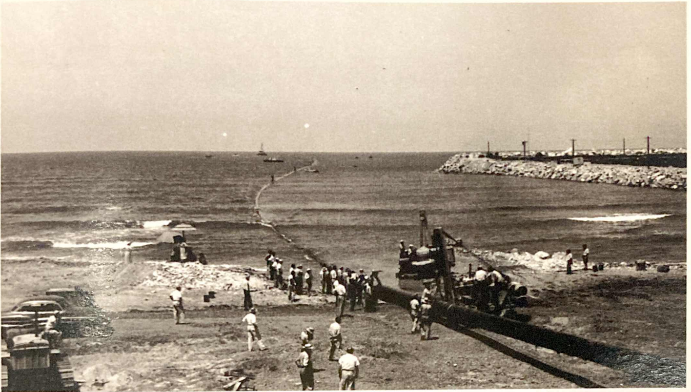
The construction of the Zahrani Terminal in 1949–1950. Courtesy of Nazih Cheikr
