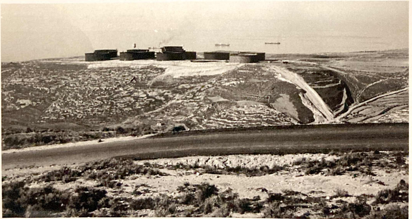
General view of Sidon Terminal in 1950. The white line coming from the hill on the right is where the pipe line is buried. Courtesy of Nazih Cheikr
